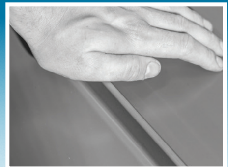
Snap the next panel in place.
