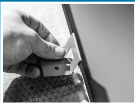
Attach the hidden clip to panel.
