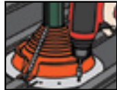
5. Fasten Retrofit to roof
