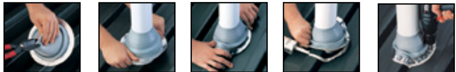
1. Choose pipe opening and trim 2. Slide over pipe 3. Form to roof profile 4. Apply sealant 5. Fasten to complete
